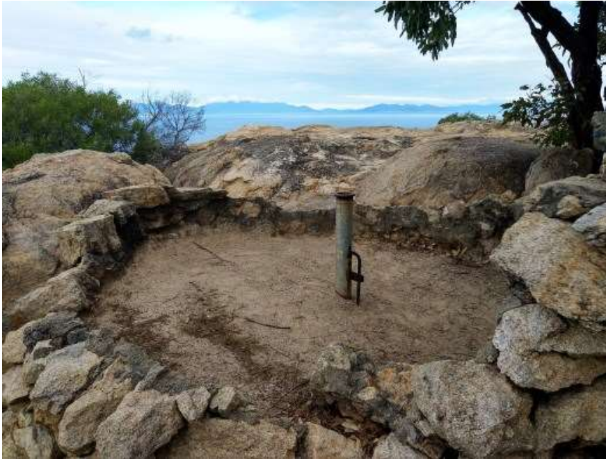
A few steel fittings and rudimentary stone enclosures are all that now remain at the Cape Edgecumbe site which, unlike the Charlies Hill site to the north, affords commanding views in all directions.
