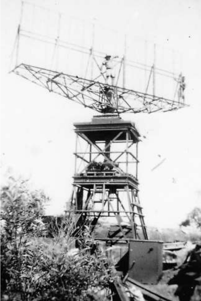
The antenna and its tower, built by the NSW Government railways in Sydney, comprised one common transmit and receive aerial that was made up of a 5-bay, 4 stacked dipole array mounted in front of a reflecting screen. The array could be rotated at 1, 1.5, 2 or 3.33 rpm (Bowen Historical Society & Museum).
